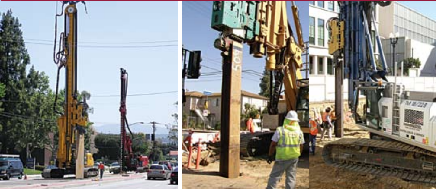
Vibrating near homes and buildings without causing damage or disturbance
