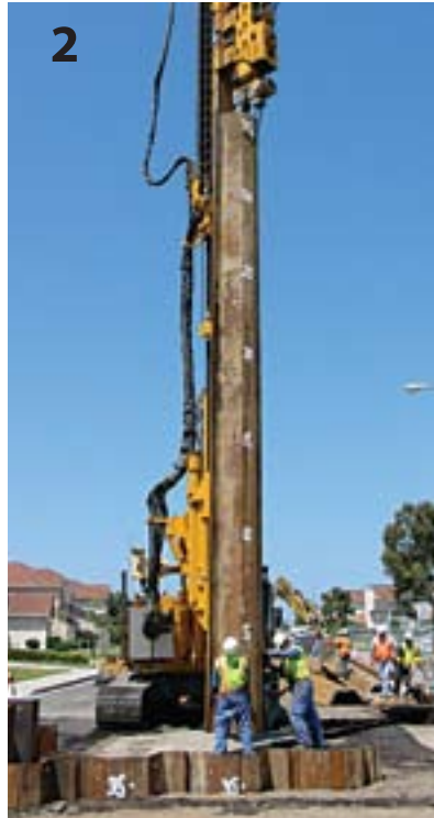
Chains position piles under the jaw
