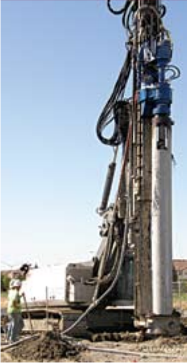
DUAL ROTARY HEAD FOR SECANT PILE
