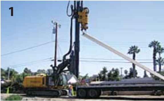
Chains on the hammer lift the pile.
