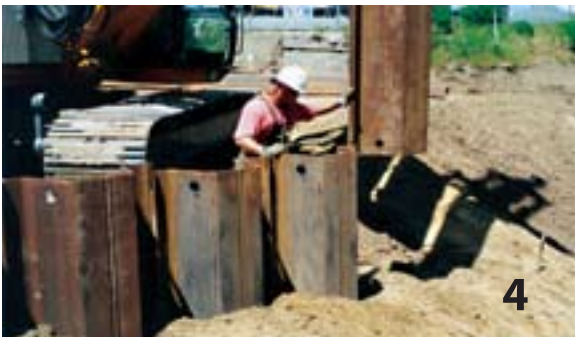
The pile is locked and is easy to handle at waist level
