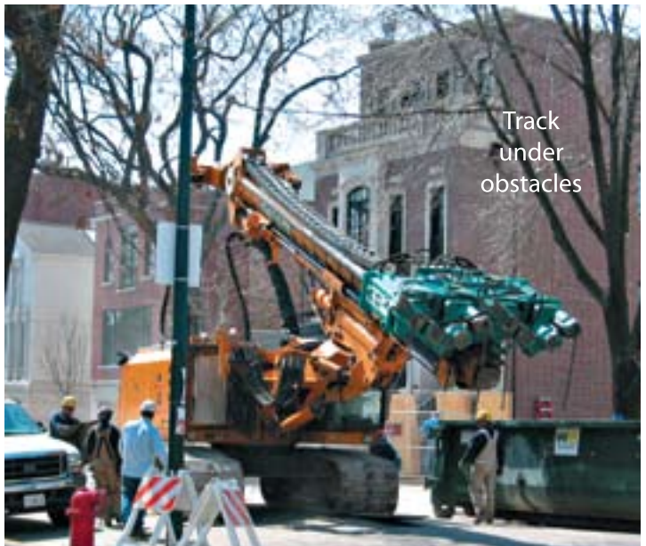
180 degree slewing of the mast
