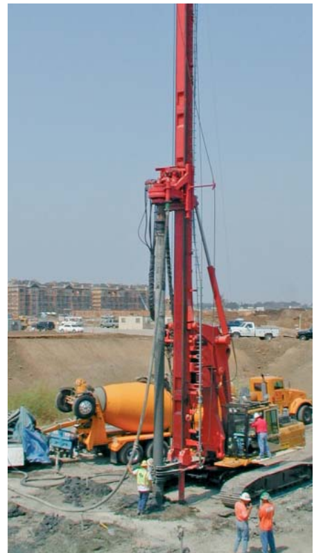
Full displacement drilling
