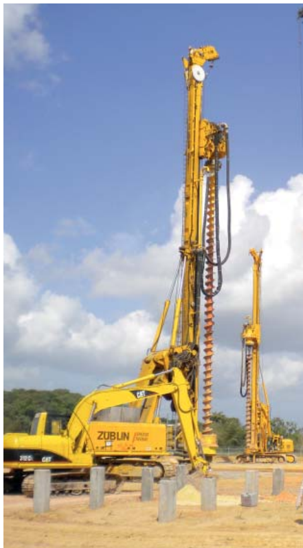
CFA drilling
