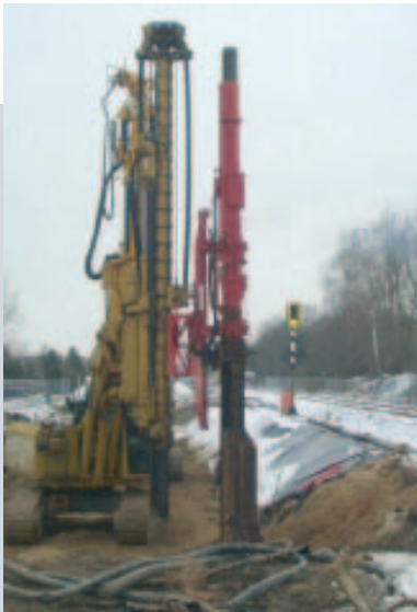
ABI - MOBILRAM with Diesel Pile Hammer D19-52 with hydraulic starting device.
