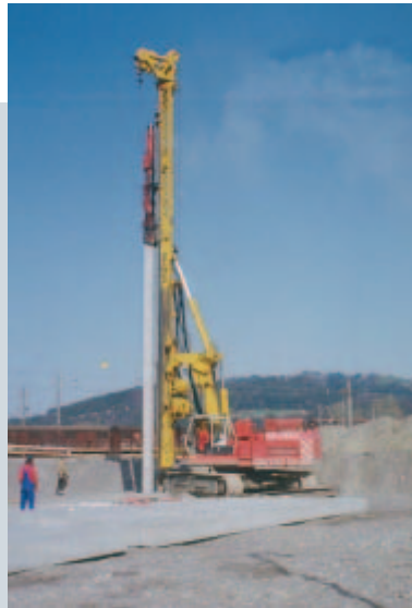
Diesel Pile Hammer attached to a DELMAG Drilling Rig RH 1413.
