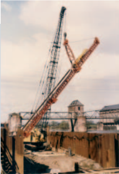
Swinging Lead for beams, pipe piles or sheet piles.
