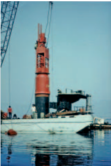
MAR-Type Lead with floating striker plate for piles up to 4.200 mm of diameter.
