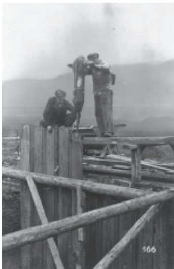
Delmag Compactor driving sheet piles (1942).
