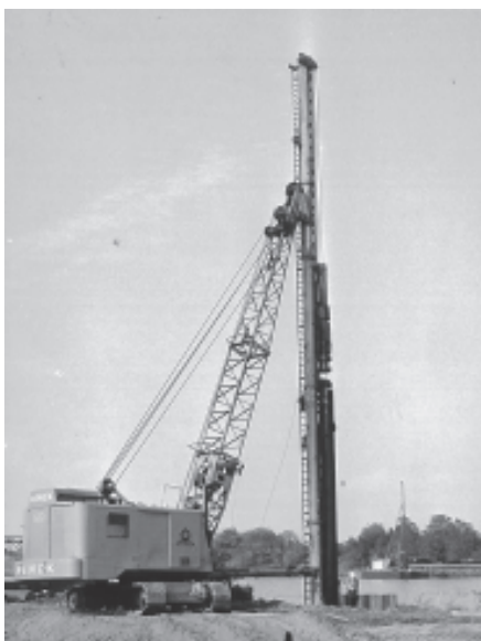
Diesel Pile Hammer attached to a DELMAG Piling Rig (1950).
