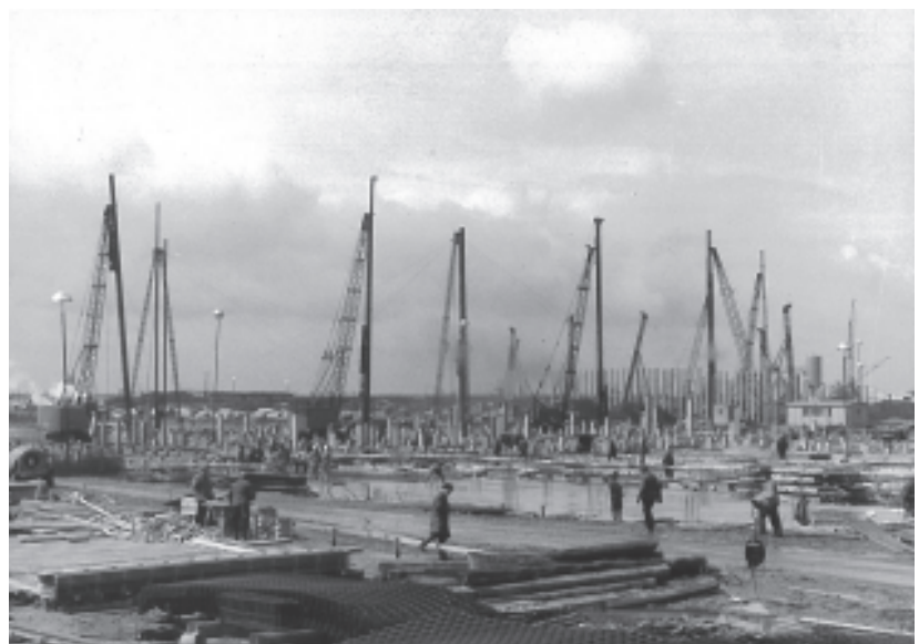
16 Delmag Swinging Leads working on a jobsite in Emden, Germany (1952).
