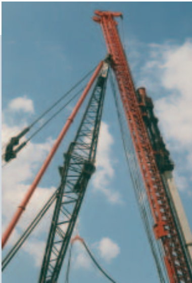
MH 37107 with Diesel Pile Hammer D 62-22.
