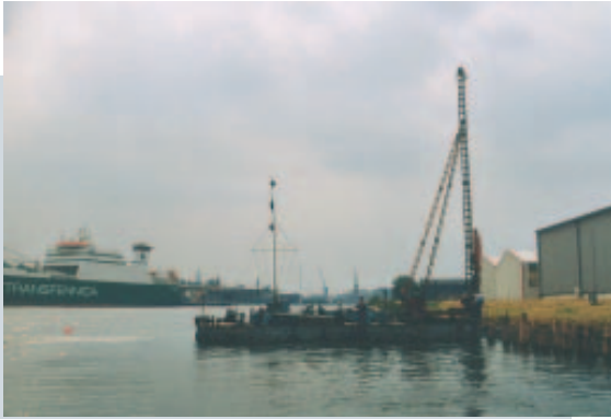
Pontoon mounted Piling Rig with D 8-22.
