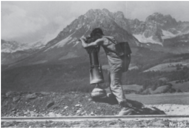
Delmag Compactor working in the mountains (1934).
