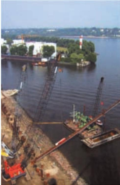
*HPH6500 on European swinging leads driving HP400 x 47m long on 1.4:1 rake (approx. 32° to the horizontal) – Hamburg, Germany*
