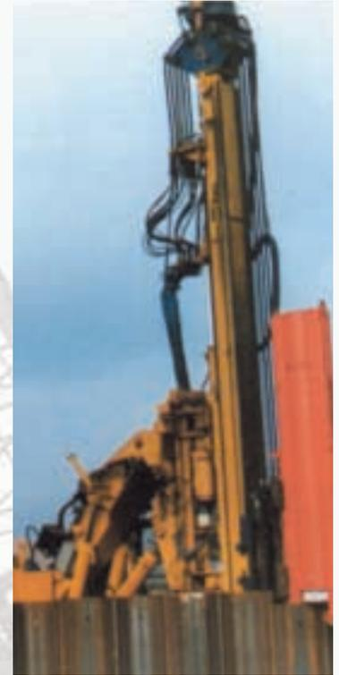
*HPH1200 on ABI Mobilram driving pairs/single steel sheet piles - UK*
