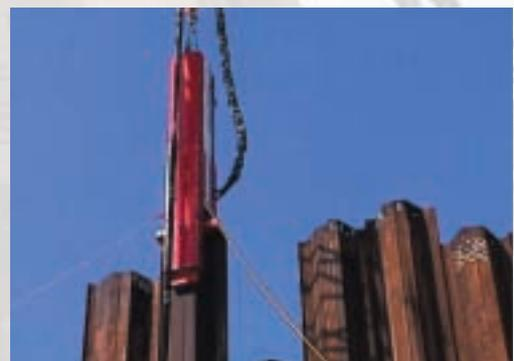
The addition of a simple spreader plate under the standard drive cap or Anvil permits all Dawson hammers to achieve almost total head coverage on any pair of sheet piles. This significantly reduces the likelihood of pile top damage in difficult driving.
