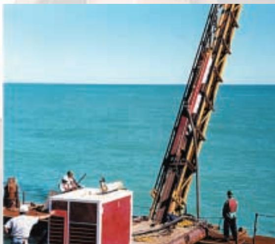
*HPH2400 fitted in 26" American leads driving 12" H-pile on a 2:3 batter – Chicago, IL, USA
