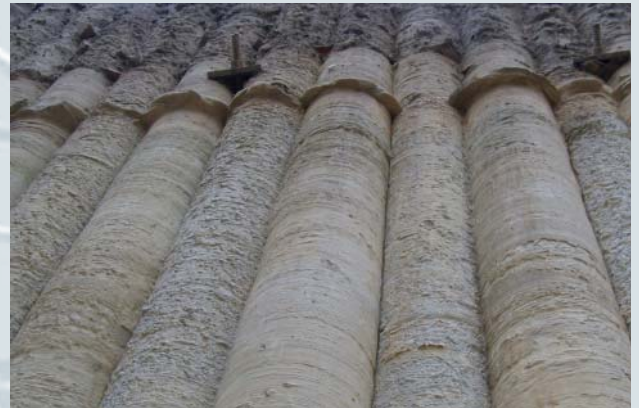
Finished exposed mixed secant pile wall
