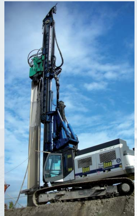
Installing cut-off wall with the fixed static moment vibrator MRZV-S
