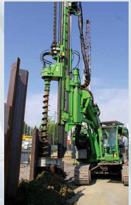
Pre-boring with auger drive MDBA
