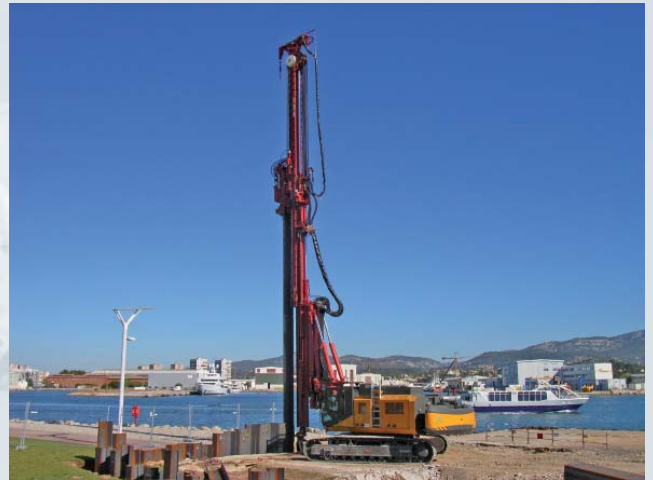
Driving U-shaped sheet piles with a variable moment vibrator MRZV-V
