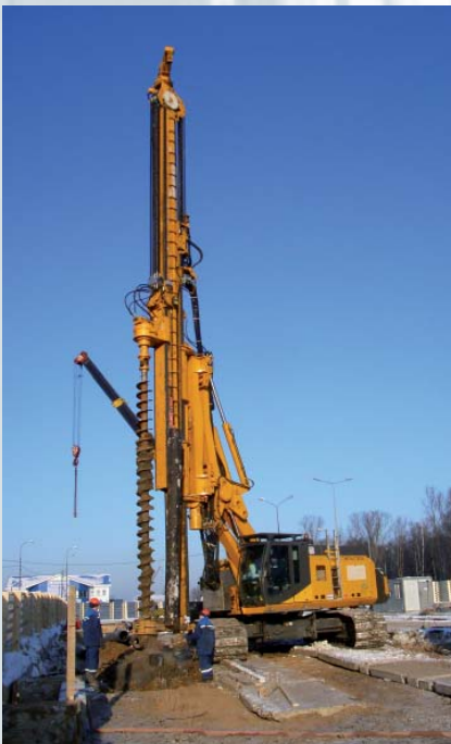
Installing CFA piles
