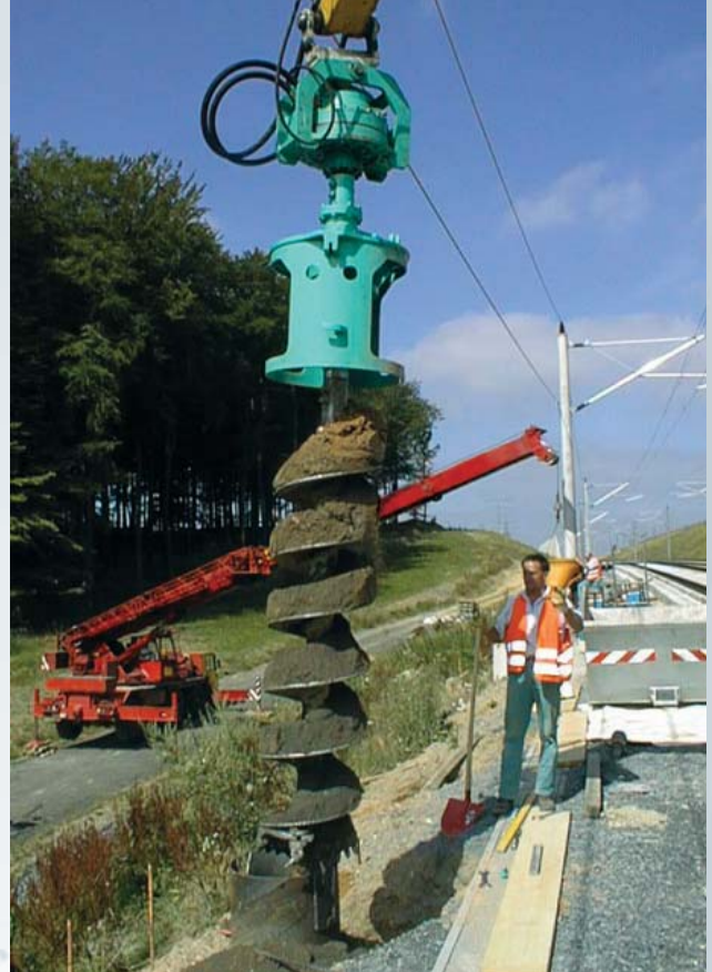
ABI auger drive with casing twister for foundation piles along rail way
