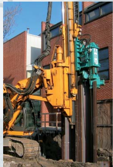
Pressing of steel sheet piles with ABI Hydro-Press-System
