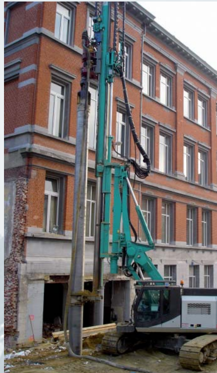
In front of the wall procedure VDW installing secant pile wall
