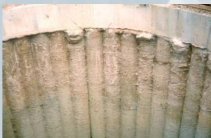
Circular cover dam done with VDW-method
