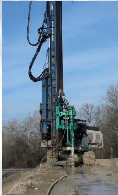
Wet Speed-Mixing with TMBA auger drive
