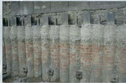
Finished wall exposed mirroring the drill through brick wall
