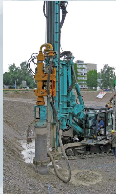
Drilling VDW piles to secure an excavation
