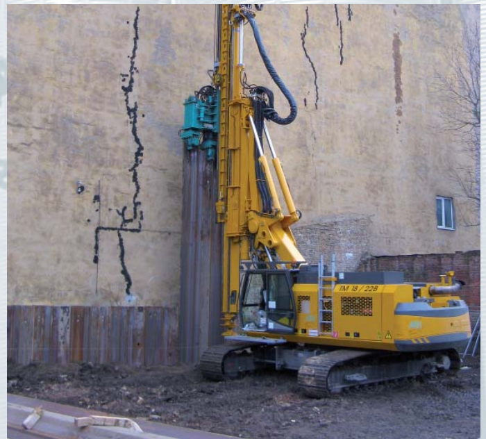
Pressing U-sheet piles panel with the HPU press direct onto an existing buildings
