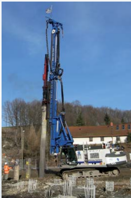
Driving tubular piles with ABI MOBILRAM-System and DELMAG diesel pile hammer
