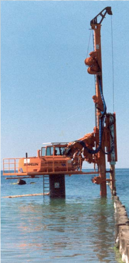
Timber pile driver off shore
