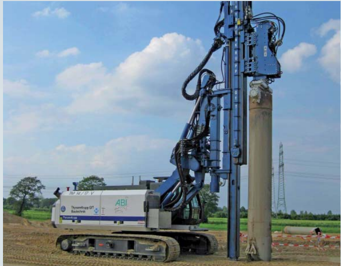
MRZV-V with casing clamp assembly driving geotextil columns
