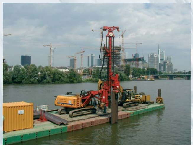
Pile driving from a barge
