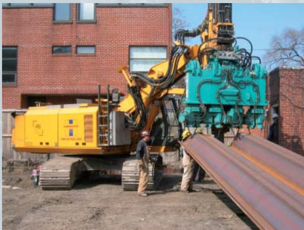
Pitching the profiles with the HPZ press
