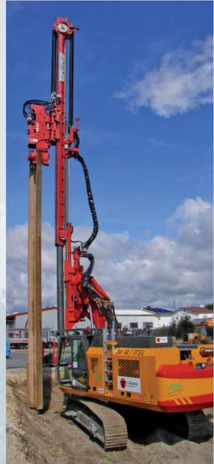
ABI MOBILRAM-System - telescopic leader mast positioning of steel sheet piles
