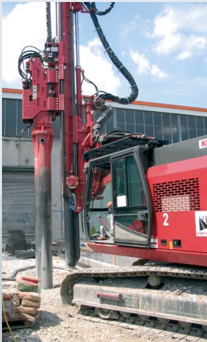
Vibropile installation with lost plate
