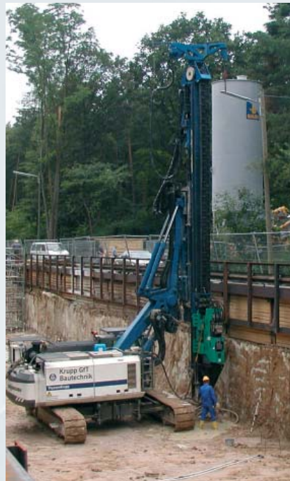
Placing soft gel injection tubes with MRZV-V and mandrel
