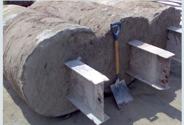
Exposed mixed element with reinforcement installed with the Triplemix auger drive TMBA
