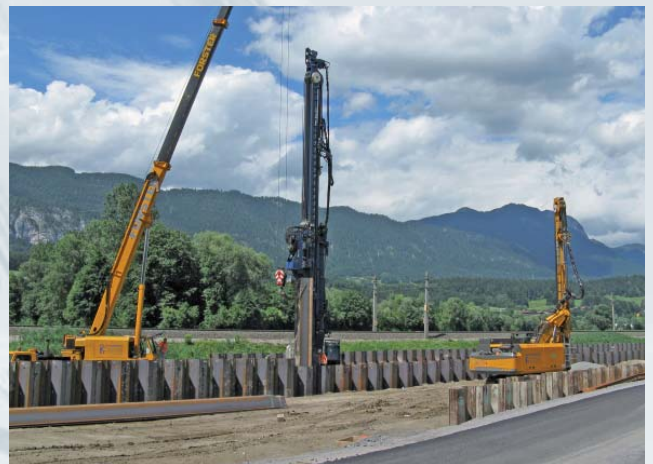
Driving steel sheet piles, piles are fed by crane
