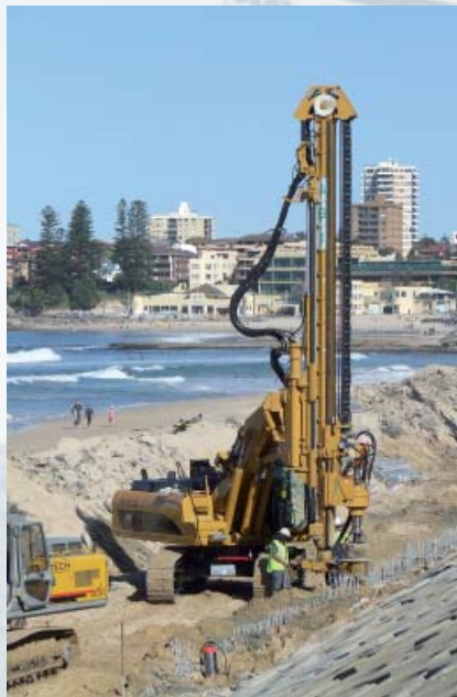
Installing cast-in-situ piles with ABI MOBILRAM-System and auger drive MDBA
