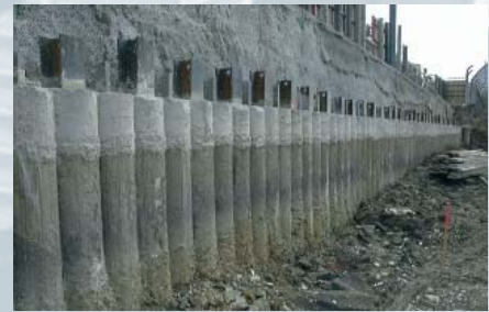
Straight wall with H-beam reinforcement
