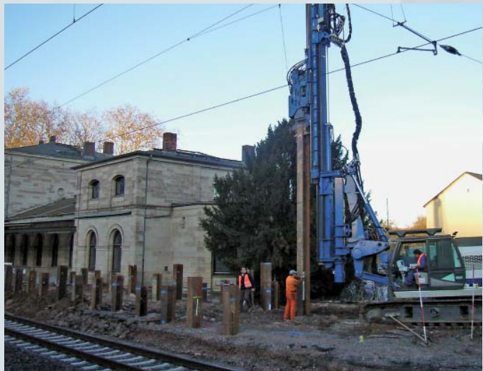
Driving H-beams for foundation
