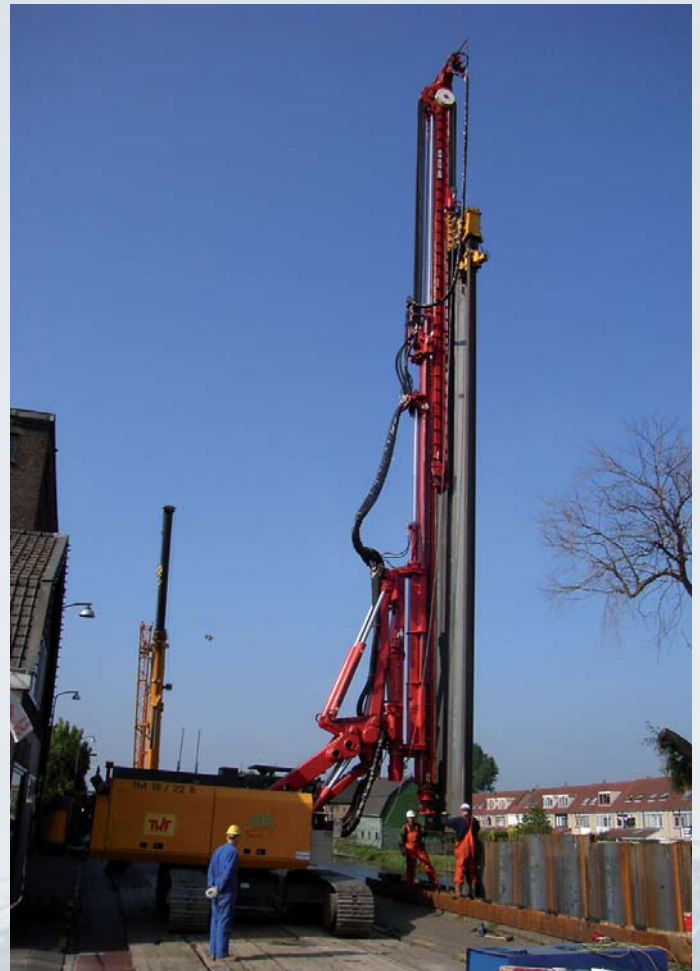
Threading Z-shaped sheet piles in interlock of previous pressed sheet panel
