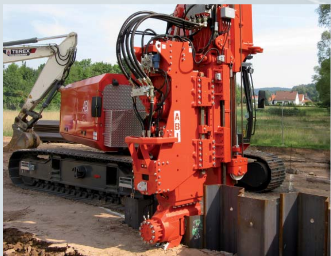
Driving sheet piles to a maximum depth
