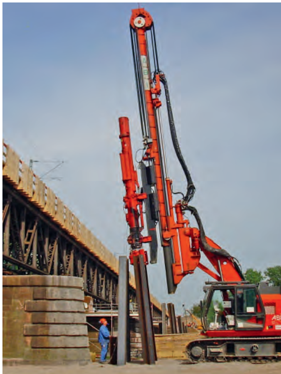
Impacting H-beams with DELMAG diesel pile hammer. With the DELMAG formula the load bearing capacity of the soil can be prooved.
