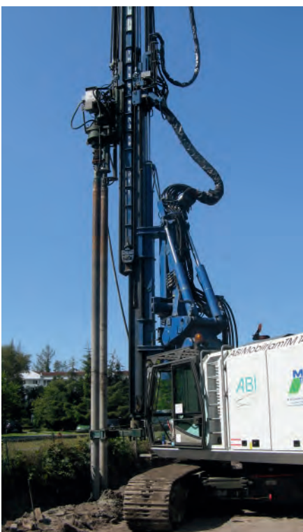
To achieve more efficiency the soilmixing procedure can be carried out as twin- or triplex version, mixing two or three piles simultaneously.
