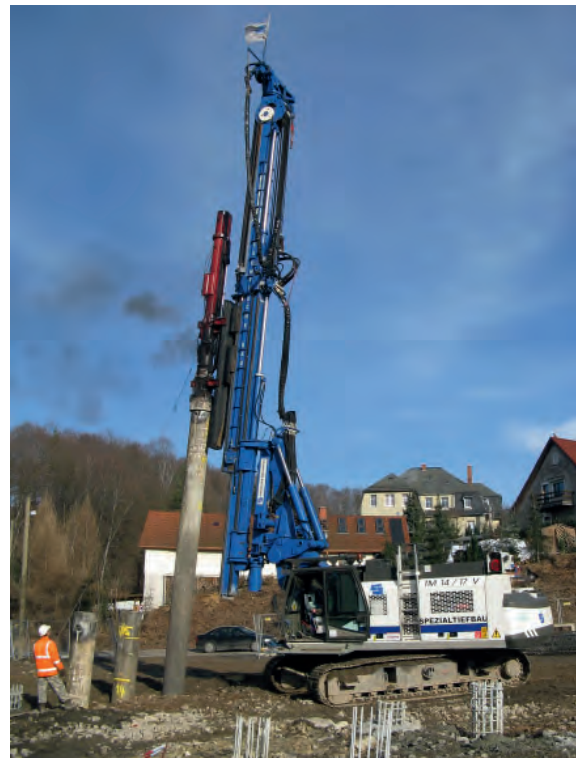
Driving casings with DELMAG diesel pile hammer.
