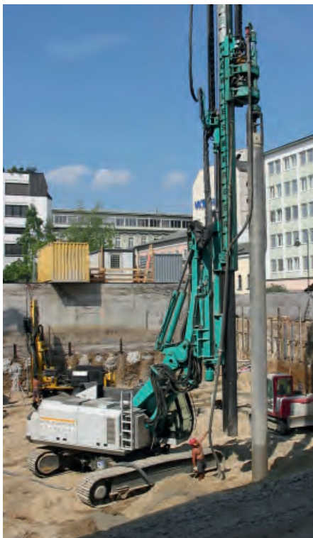
VDW drilling: with the VDW double auger head system cased single piles as well as secant pile walls can be installed. The drilling is carried out in one step, after drilling down concret is pumped during withdrawal.
