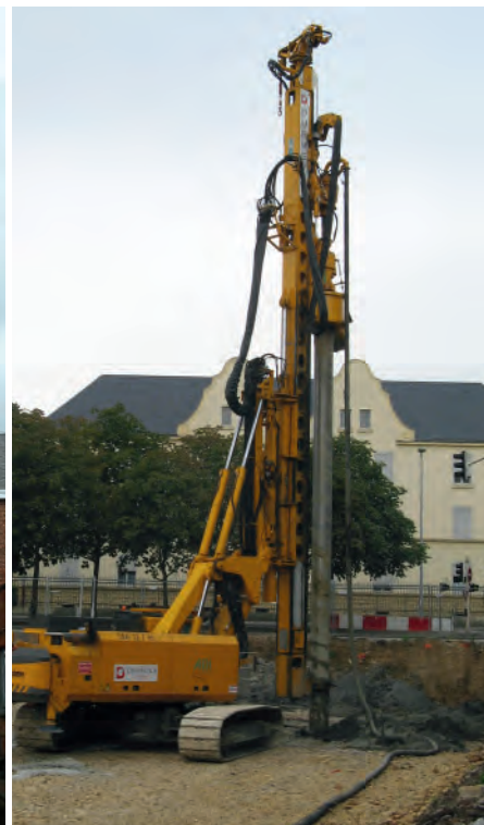
Double auger head system DH 18: works similar as VDW, but the auger heads are separately moveable. It enables the auger to be withdrawn while the casing ist staying in the ground.
