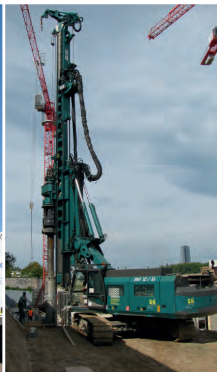
Kelly drilling: the machine is equipped with a kelly winch. The casing is drilled as deep as possible first and then drilled out with the auger. This process is being repeated till the requested depth is achieved.
