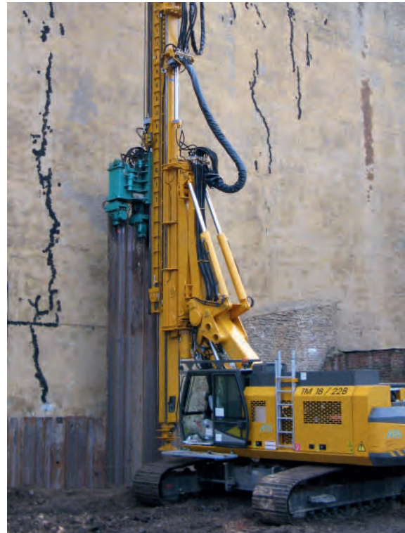
Static pressing direct in front of an existing building. In some cases the soil have to be loosened by pre-drilling before pressing.
