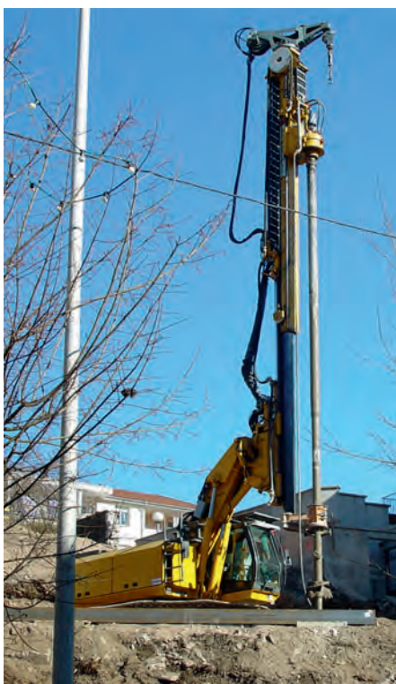
Soilmixing WSM: homogenous concrete piles are formed by mixing the existing soil with suspension while drilling and extracting the mixing tool.
