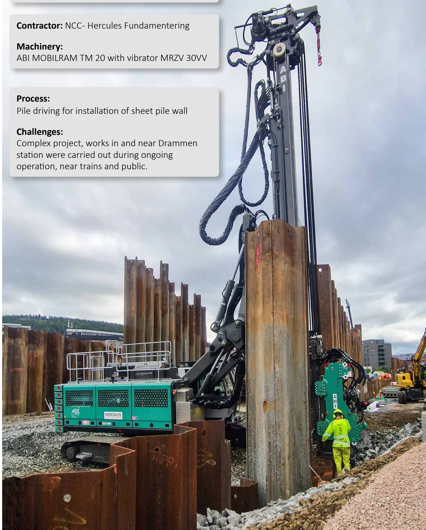
Photo: ABI MOBILRAM TM 20 with vibrator MRZV 30VV while pile driving
