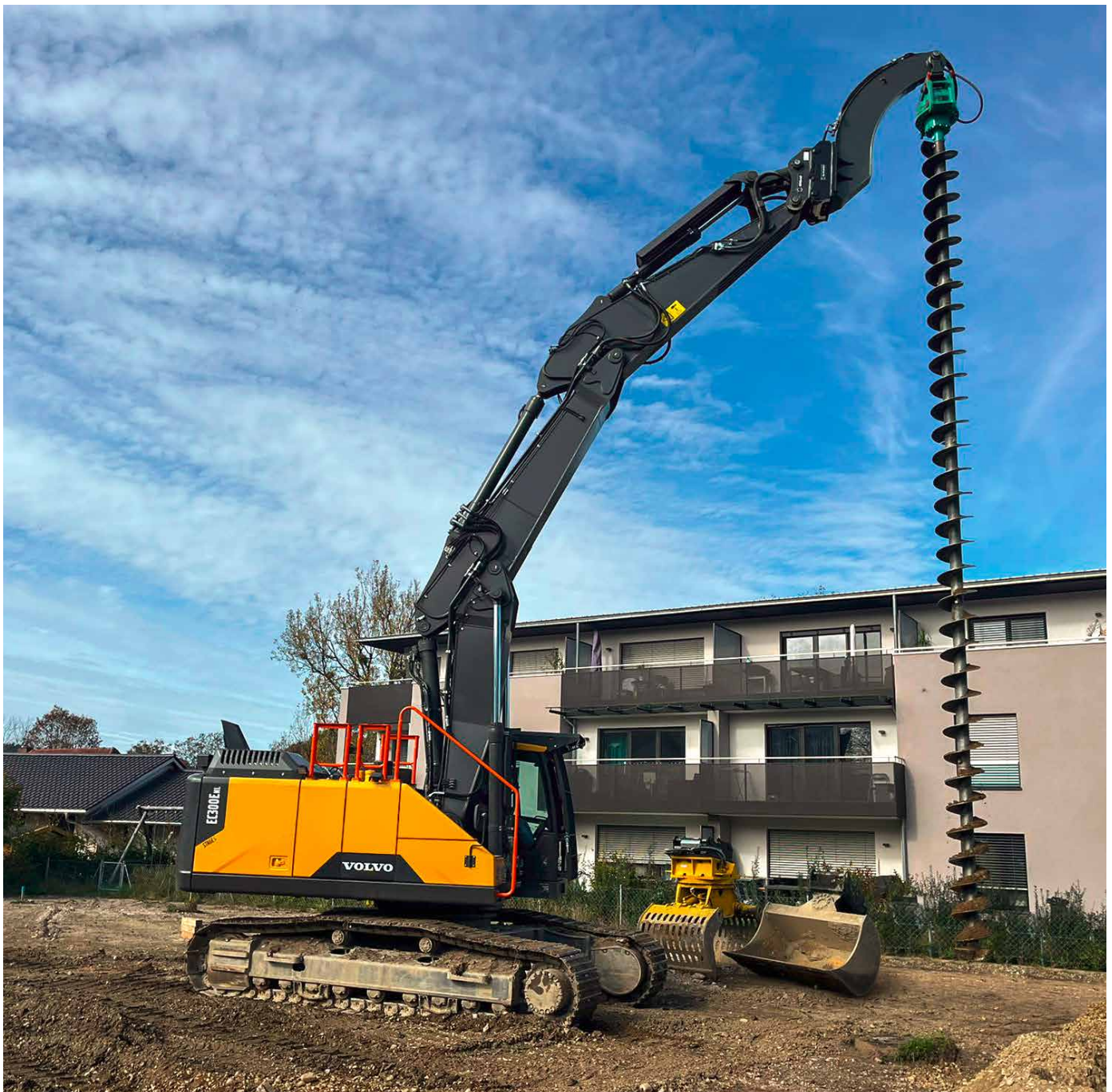
Photo: ABI auger drive BA 2200 with quick-coupling system and stick extension with 10m auger on the job site
