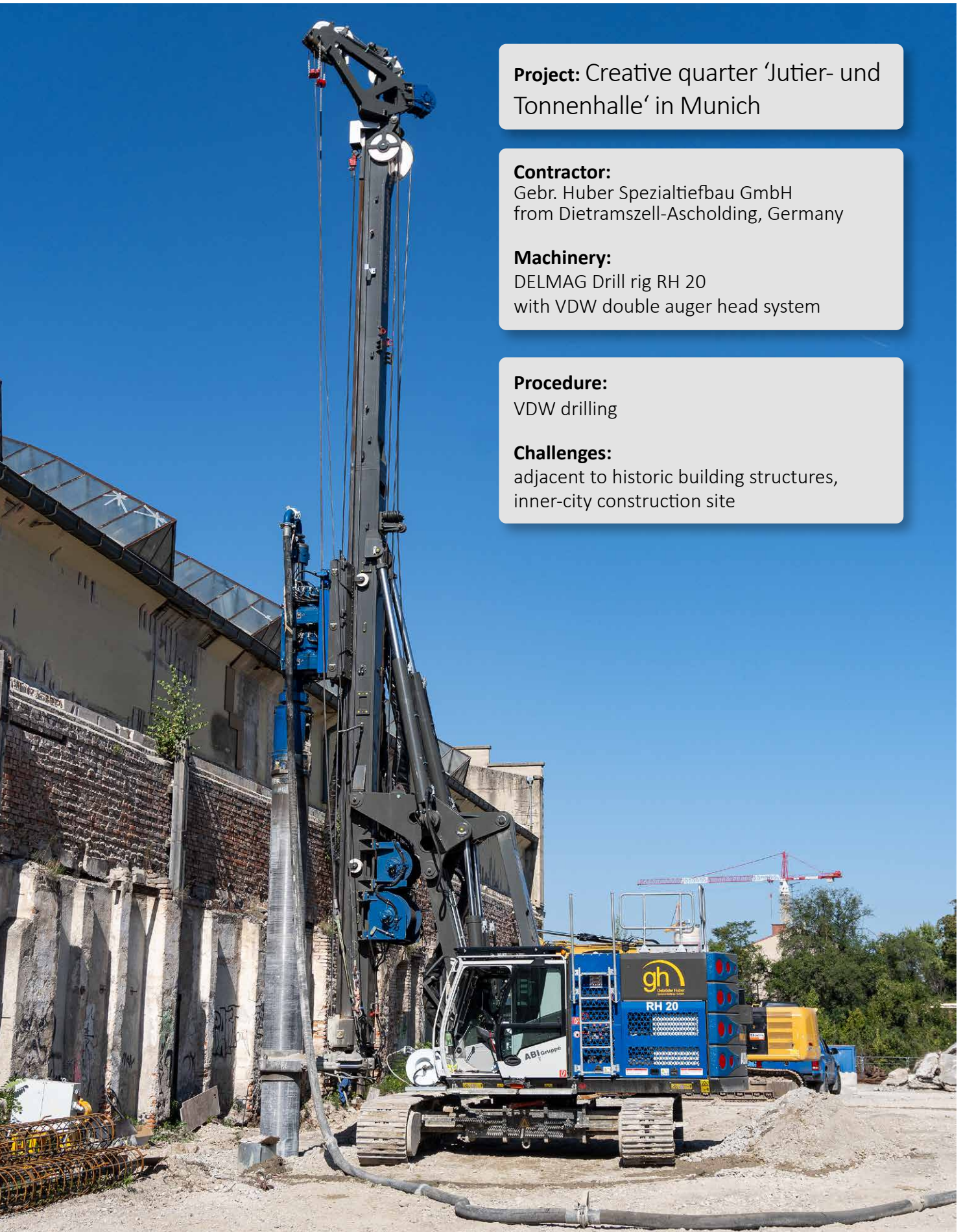
Photo: DELMAG drill rig RH 20 with VDW VDW double auger head system while installing secant pile wall
