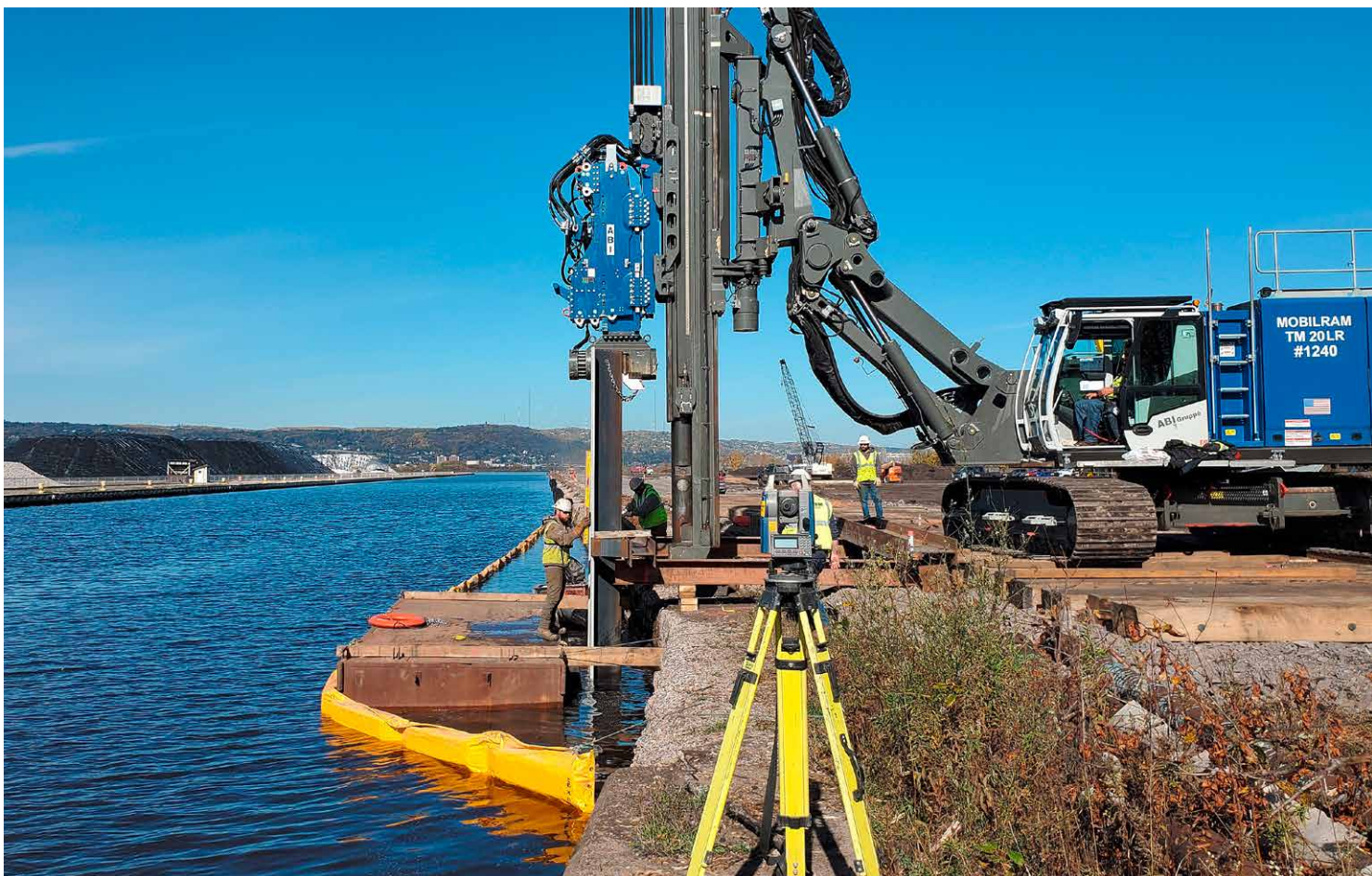
Photo: ABI MOBILRAM TM 20 LR with Vibrator MRZV 30VV on the St. Louis River, USA
