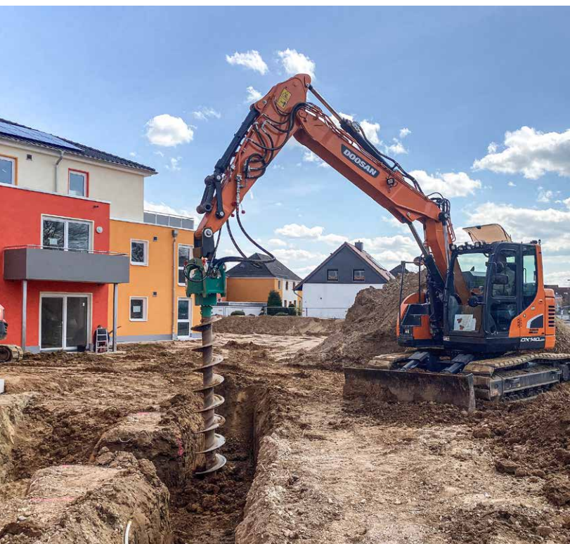
Photo: uncased drilling for a geothermal probe with the ABI excavator mounted auger drive BA 2200
