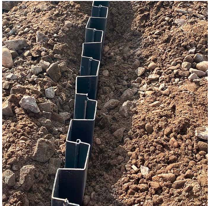
Photos: Finished measures for the harbour development at Fort William (above), Driven-in plastic sheet pile wall (below)
