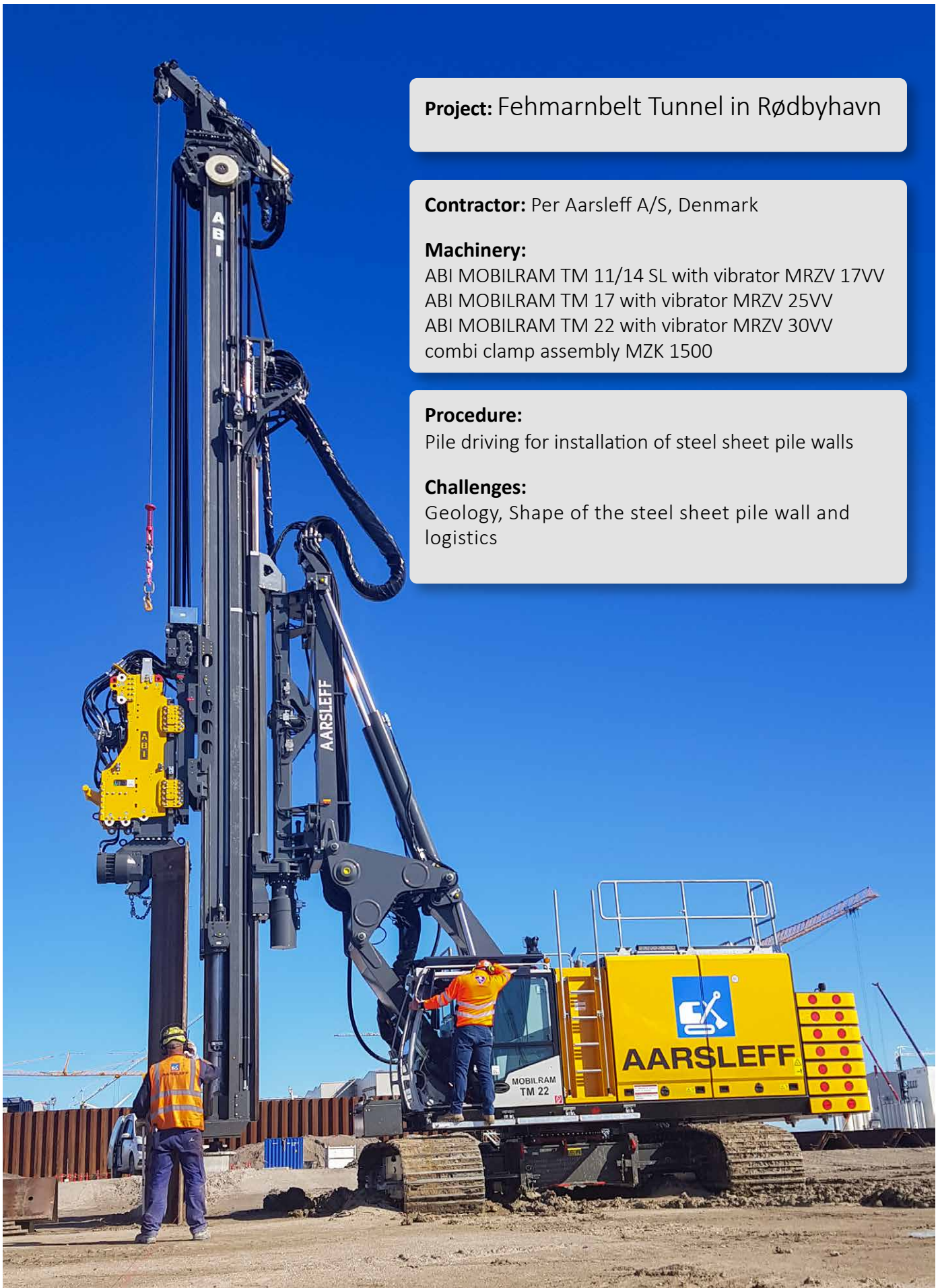
Photo: ABI MOBILRAM TM 22 with vibrator MRZV 30VV while pile driving at the job site in Fehmarnbelt-Tunnel
