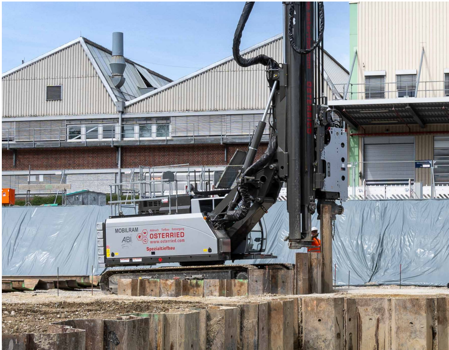
Photos: ABI MOBILRAM TM 13 with vibrator MRZV 16VV while pile driving at the job site in Munich
