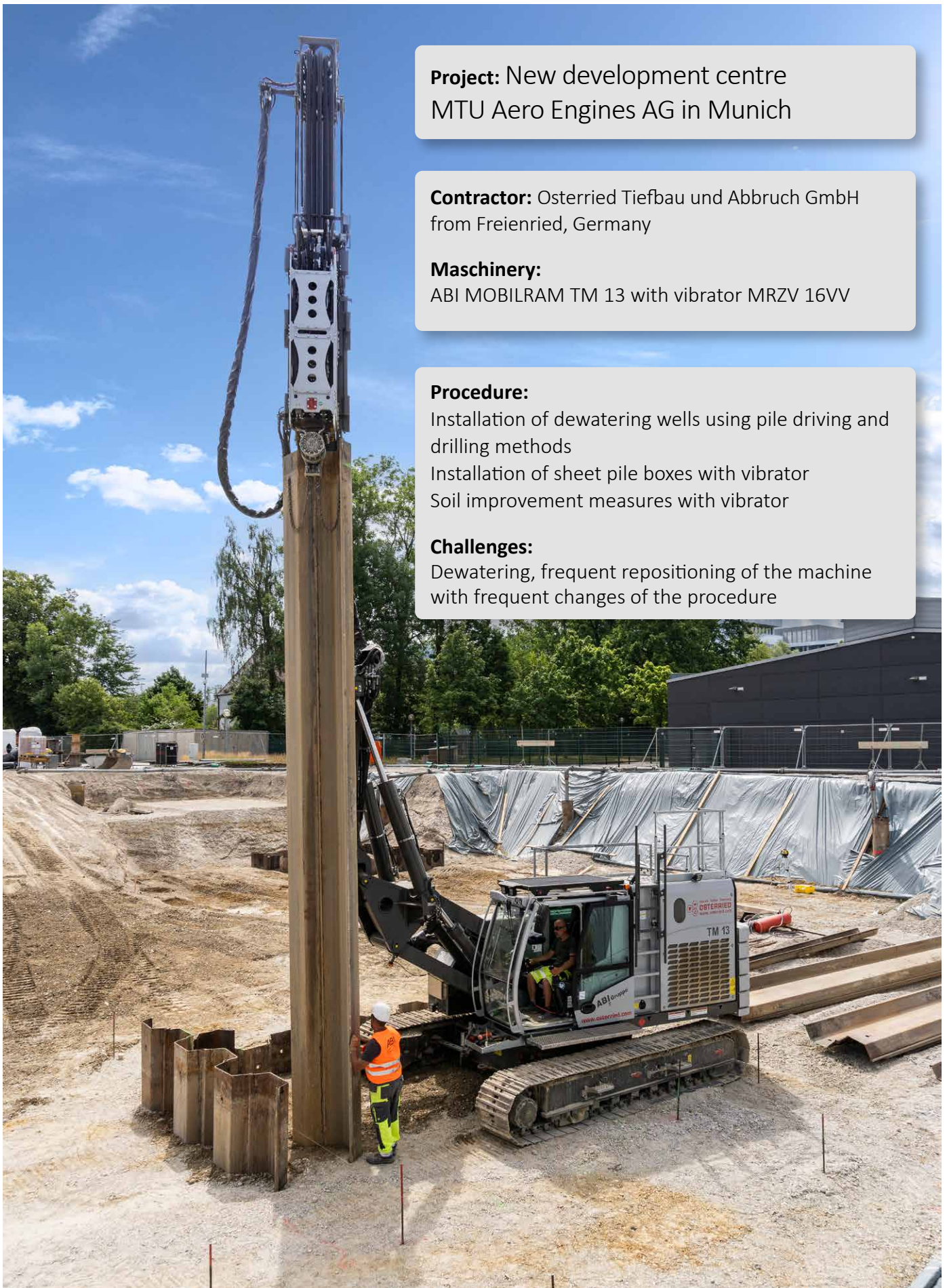
Photo: ABI MOBILRAM TM 13 with vibrator MRZV 16VV while driving U-shaped steel sheet piles
