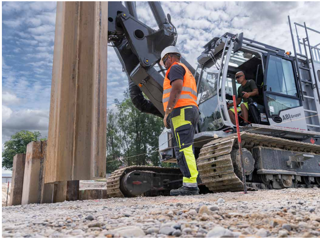
Photos: ABI MOBILRAM TM 13 with vibrator MRZV 16VV while pile driving at the job site in Munich
