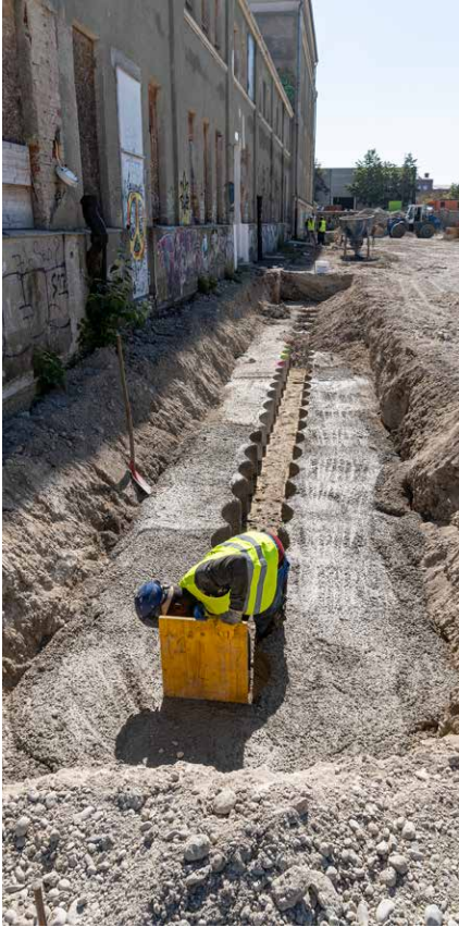
Photo: Template for a secant pile wall
