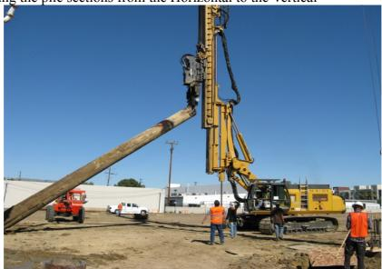
This is possible for both types of piles, King piles and fill piles. The sheet piles will be taken as pairs or triples to speed up the operation.
