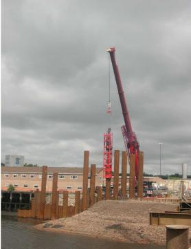
In rather high blow count soil formation we offer our Delmag diesel pile hammers with drive cap to suit the dia. Of the tubular King piles.
