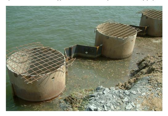
The hard driving of the second section of the tubular piles will be done by the Impact hammer hanging of suitable size crane.
