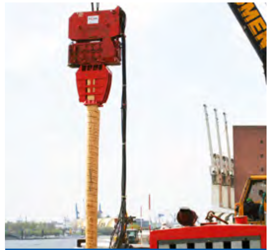
30HFV Vibrodriver driving wooden piles at the entrance of the Marina, Hamburg-Germany.
