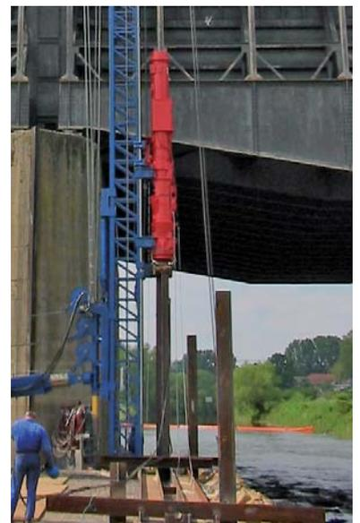
Hanging lead MH 6204 with diesel pile hammer D30-32 at the Dortmund -Ems channel in Germany
