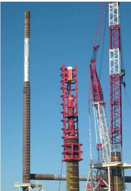
DELMAG diesel pile hammer D200-42 driving 84" pipe piles in Caspian Sea
