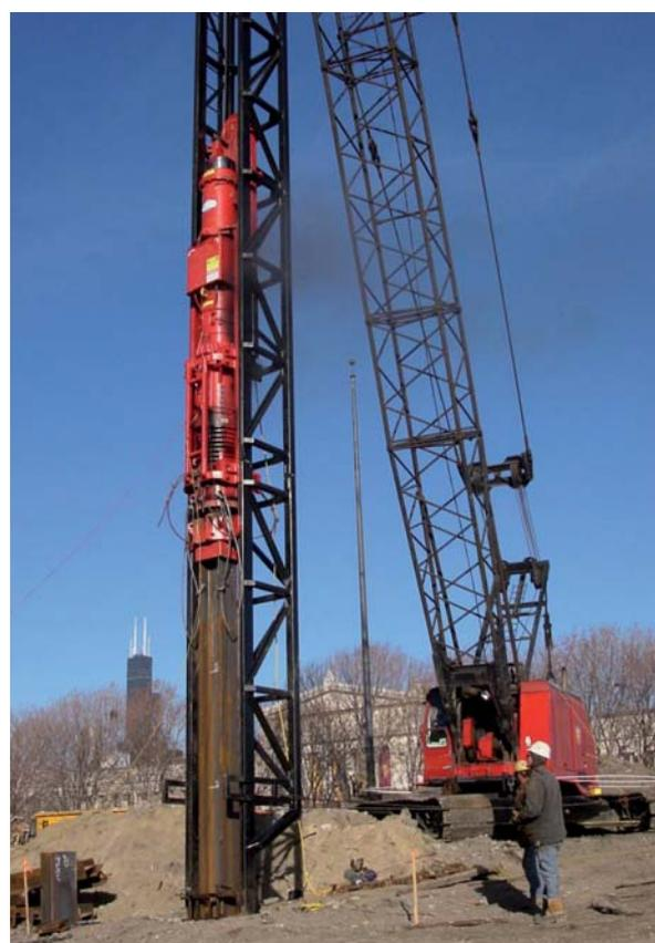
Swinging lead MU 6200 with DELMAG diesel pile hammer D36-32 in the USA
