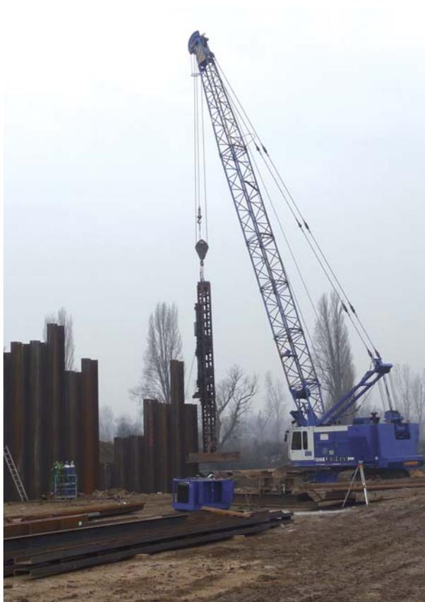
Swinging lead MS 3003 with DELMAG diesel pile hammer D25-32 in Germany
