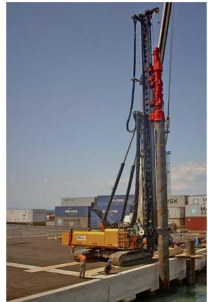
DELMAG diesel pile hammer D46-32 on piling rig BANUT 655 in Slovenia
