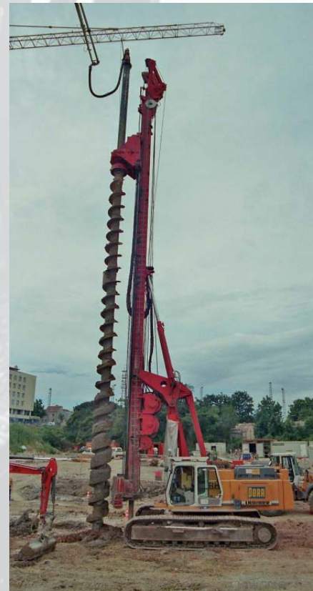
CFA drilling with a hollow auger and kelly extension
