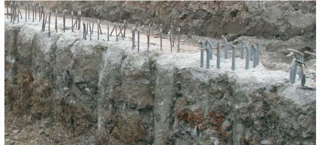
Secant pile wall with reinforcement
