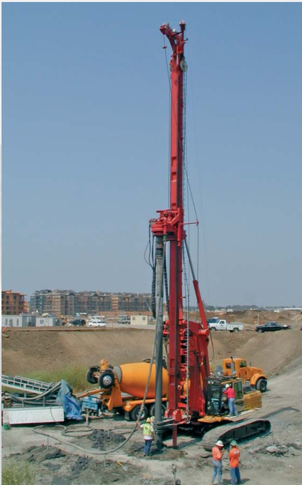
Full displacement drilling
