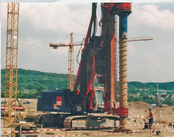
Part displacement drilling
