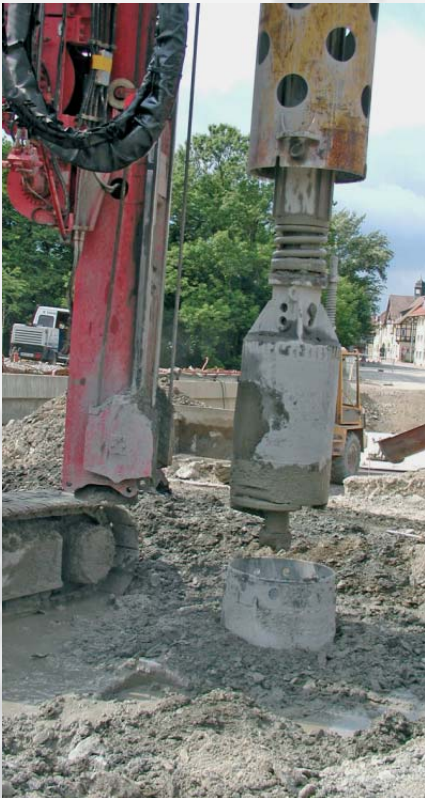
Drilling bucket for working in water saturated soils
