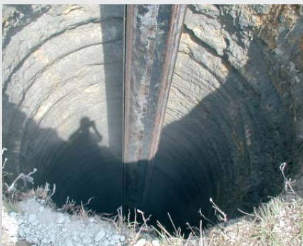
Drilling without casing in rock formation
