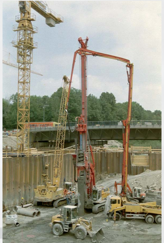
Installation of foundation piles with the DDK system (dual rotary head)
