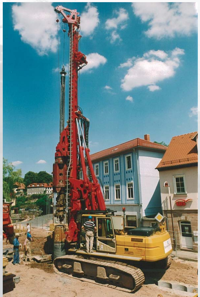
Installation of a secant pile wall using a drilling pattern
