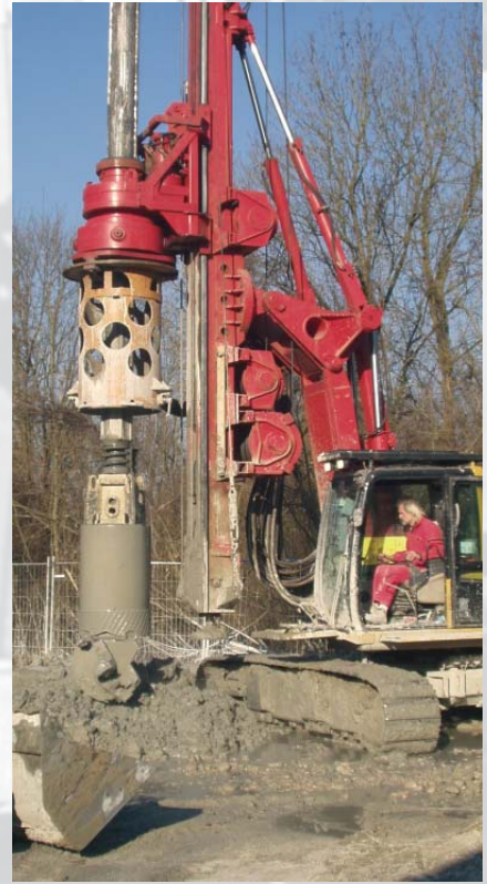
Cleaning the drilling bucket
