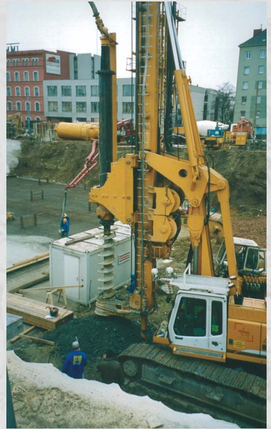
Drilling with continuous flight auger (CFA) and kelly extension
