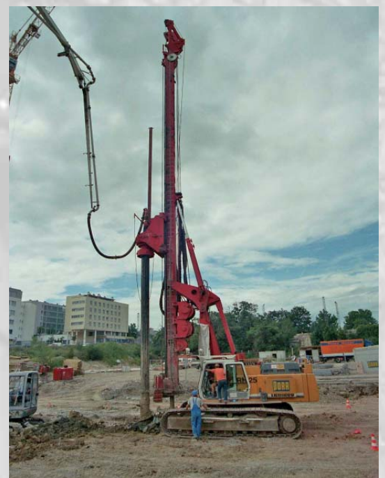
Kelly extension for maximum drilling depth with continuous flight auger
