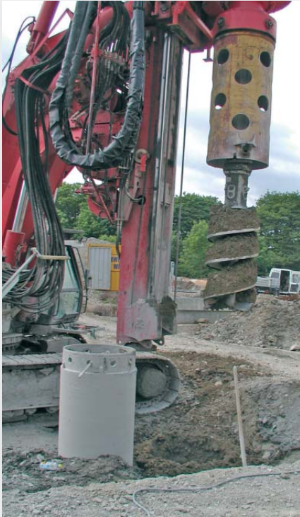
Auger filled with spoil is pulled out of the casing
