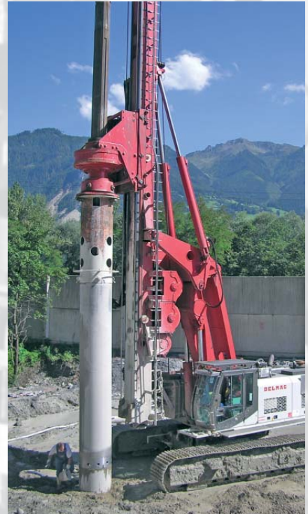
Installation of double wall casing
