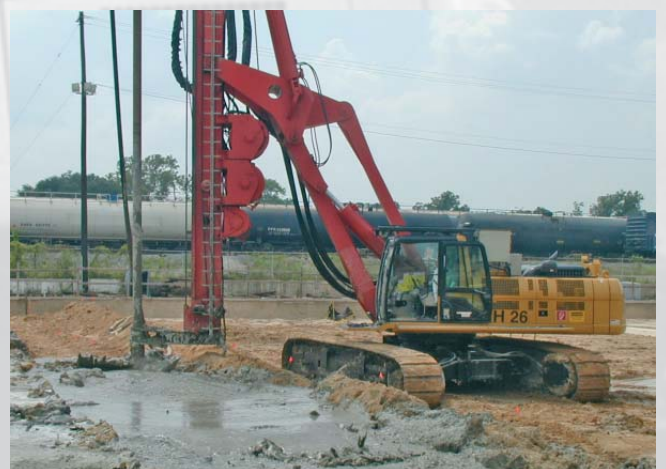
Soil mixing application WSM (Wet Speed-Mixing)
