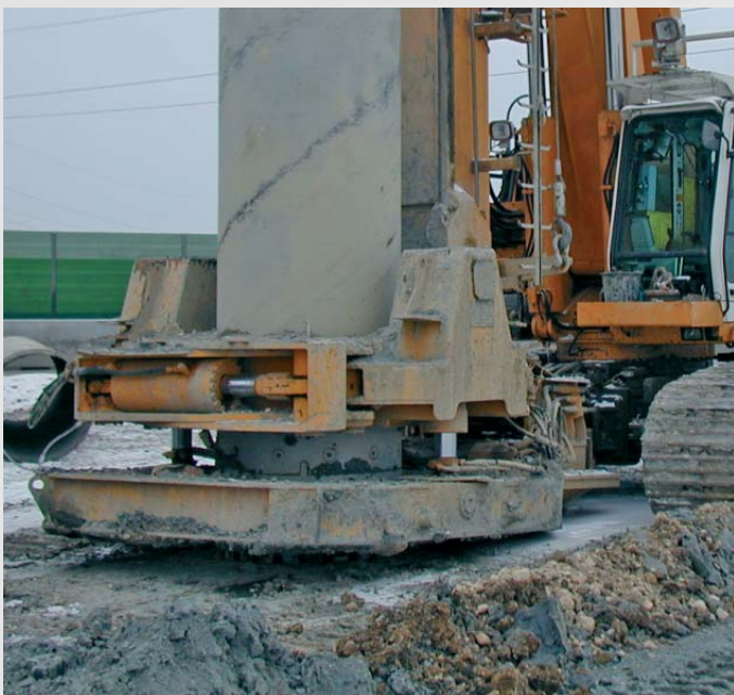
Casing oscillator for installation and extraction of casings
