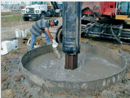
Drilling with support fluid
