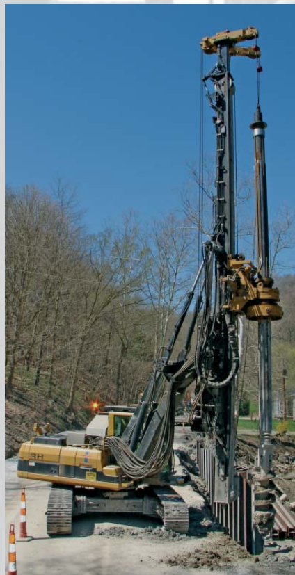
Kelly drilling without casing
