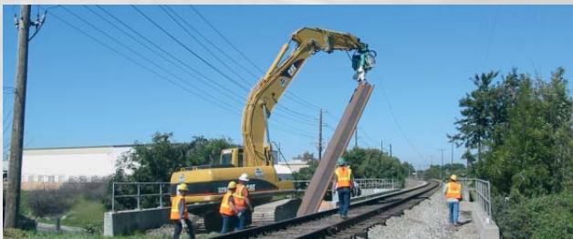
Pitching the sheet with the vibrator, safe and fast
