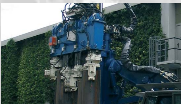
HPZ during pressing, centre pairs of sheet piles are pushed down
