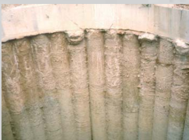
Circular cover dam done with VDW-method
