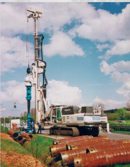
Kelly drilling with ABI fixed leader mast SM 9/10 with extra long reach
