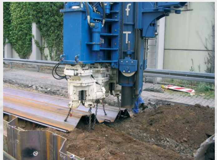
Pitching Z-shaped sheet piles with HPZ-Press
