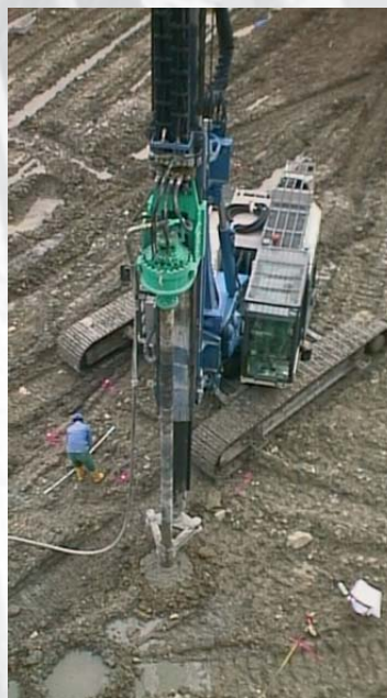
Wet Speed-Mixing with MDBA auger drive
