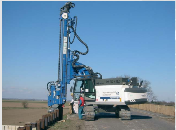
MRZV-V on telescopic leader mast TM 10/12,5 driving sheet piles
