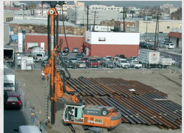
Ground release drilling for soldier beam wall in Los Angeles (USA)
