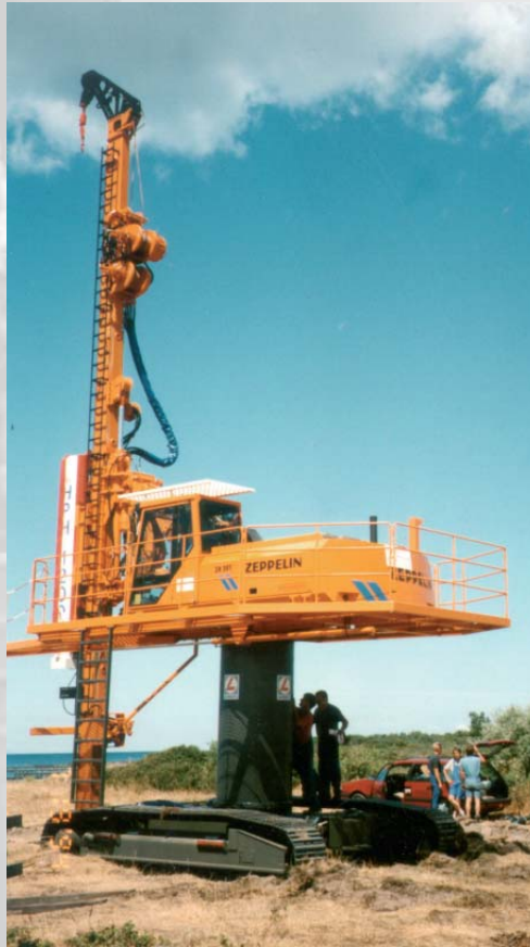
Timber pile drive on shore
