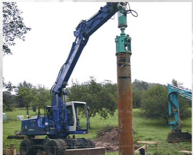
Cased drilling with BA 2250 and casing
