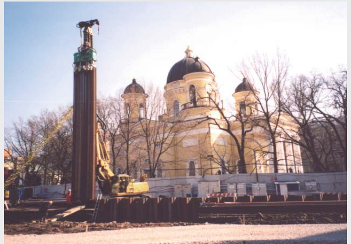
HPU pushing sheet piles in St. Petersburg (Russia)
