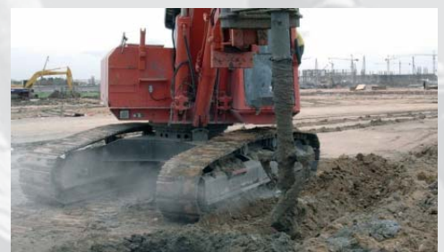
Dry Speed-Mixing in Thailand as ground improvement
