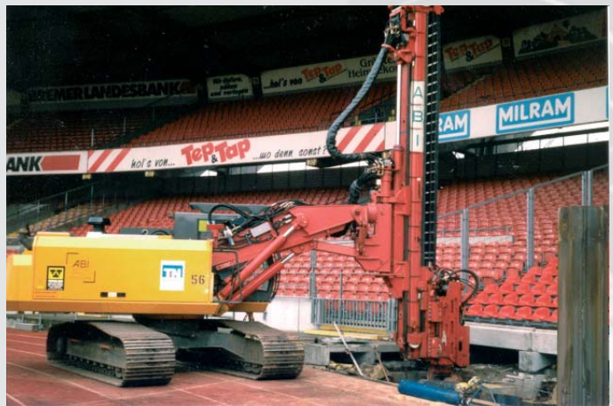
MRZV-V driving sheet piles in a football stadium in Bremen (Germany)
