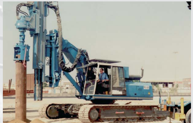
Cased drilling using MDBA and casing turn device on ABI MOBILRAM-System
