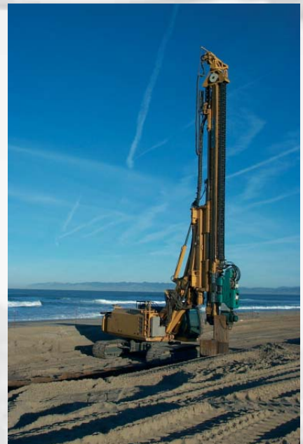
Driving sheet piles as preparation for soil exchange
