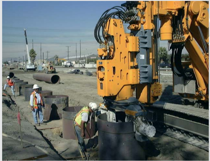
MRZV-V with casing clamp assembly to drive pipes in Los Angeles (USA)
