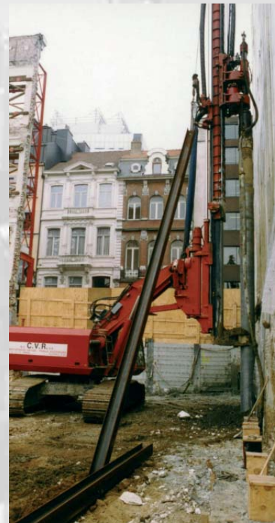
During extraction the re-inforcement is pulled up
