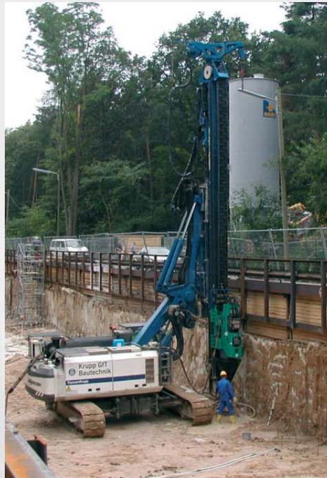
Placing soft gel injection tubes with MRZV-V and mandrel
