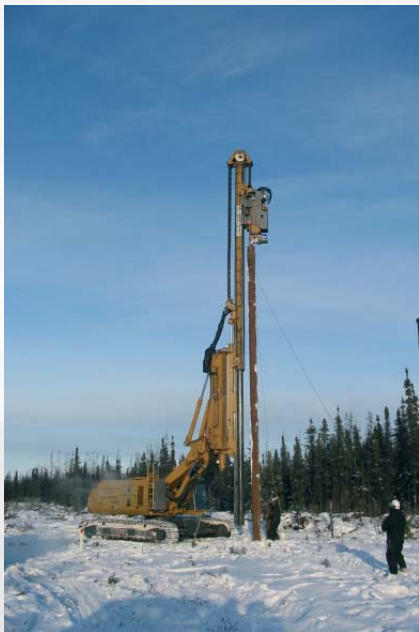
Driving foundation pipe piles
