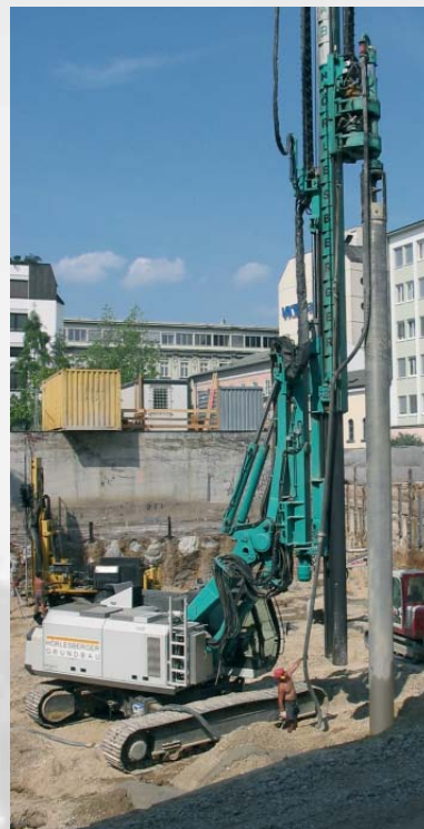
In front of the wall procedure VDW installing secant-pile wall
