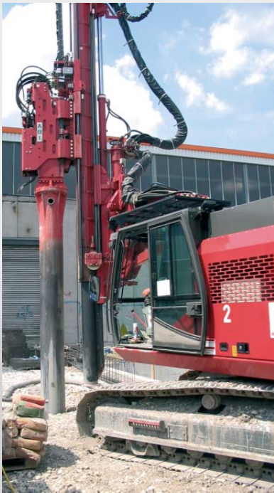
Vibropile installation with lost plate
