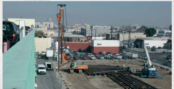
Driving H-beams in pre-bored holes on site in Los Angeles (USA)
