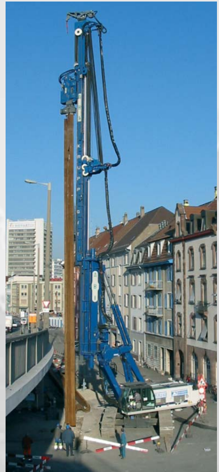
ABI MOBILRAM-System - telescopic leader mast TM 20/25 with vibrator MRZV -V
