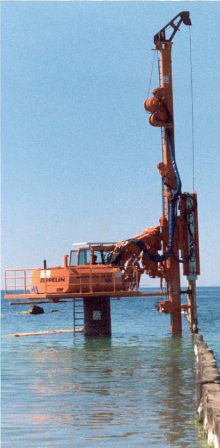
Timber pile driver off shore
