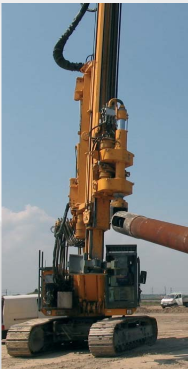
ABI MOBILRAM-System setting up casing and auger tool
