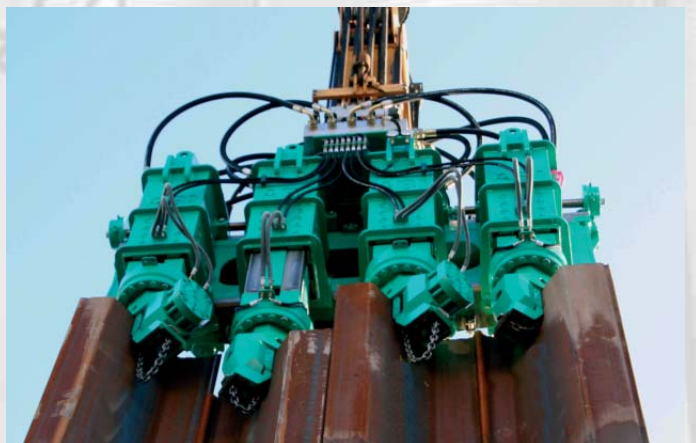
HPZ 500-720 with clamped and Z sheet piles during pressing operation
