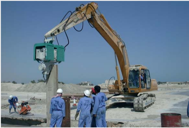
Driving sheets in sandy soils
