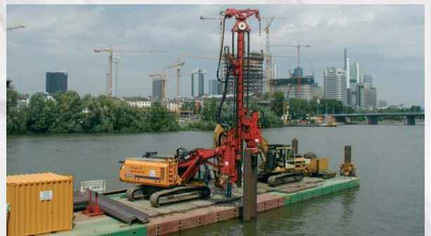
Test pile driving from a barge in Frankfurt am Main (Germany)
