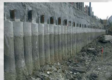
Straight wall with H-beam reinforcement
