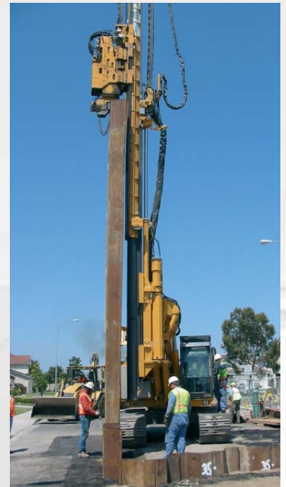
Clutching sheet piles
