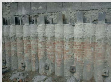
Finished wall exposed mirroring the drill through brick wall
