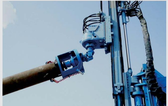
Casing and auger raised and lowered with 90 degrees cardanic joint
