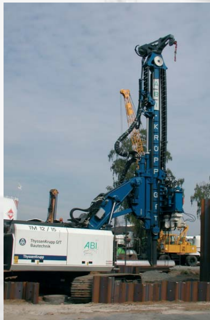
Vibration-free piling and extracting Hydro-Press-System type HPZ
