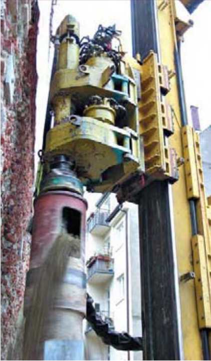
DUAL ROTARY HEAD FOR SECANT PILE
