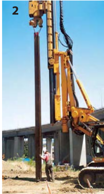
The attachment lifts the pile.
