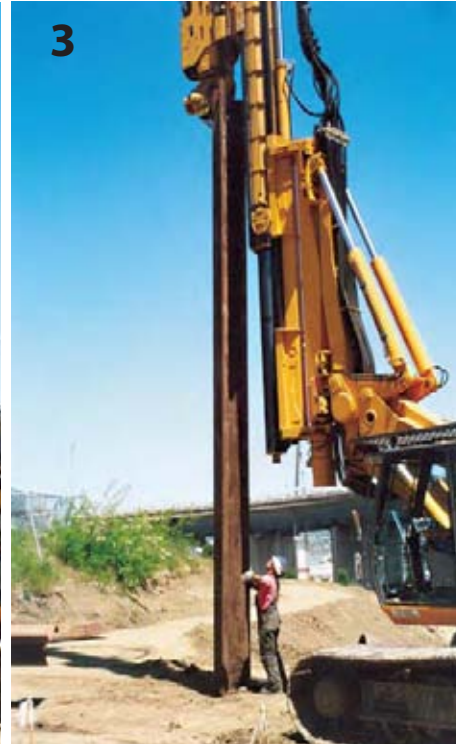
The jaws lock the pile to the rig.
