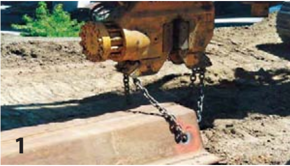
Chains on the hammer lift the pile.
