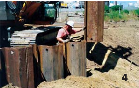
The pile is locked and is easy to handle at waist level.
