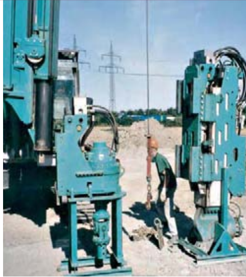
The docking system allows swapping of attachments within 5 minutes
