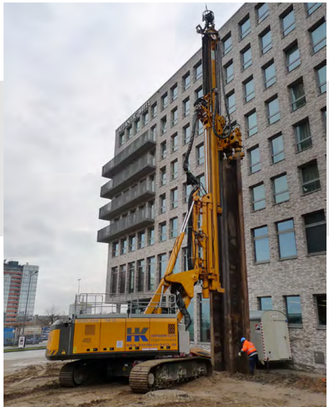
Static pressing directly in front of existing buildings. In some cases the soil must be loosened by pre-drilling before pressing.
