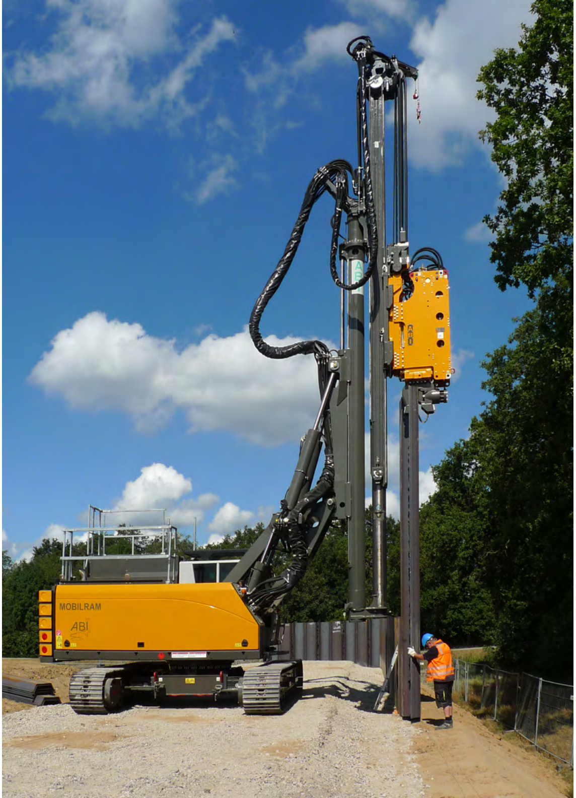
A classical application for the ABI MOBILRAM-System with vibrator: The installation of a sheet pile wall.
