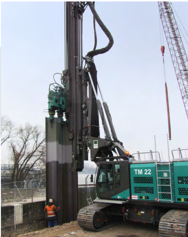
Using the Hydro-Press-System HPZ four steel sheet piles are pressed in a step sequence into the ground.
