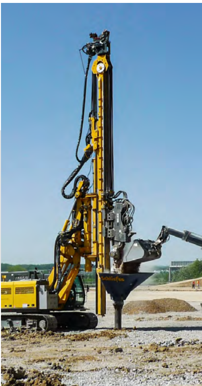
Increasing the load bearing capacity of the ground installing gravel piles.
