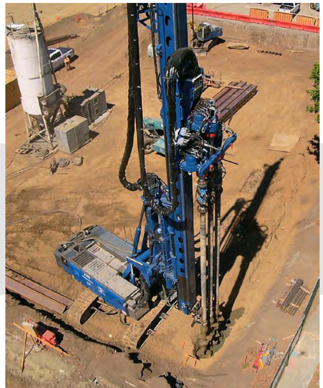
Soil mixing with the Triplemix auger drive. In one step three overlapped mixed piles are installed.
