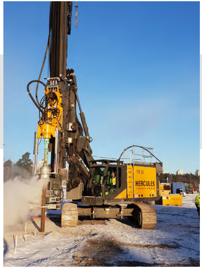
In hard, rocky soils down-the-hole hammers (DTH) are used for drilling.
